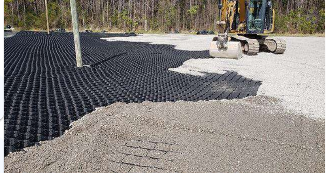
Geocell installation at road construction project site
