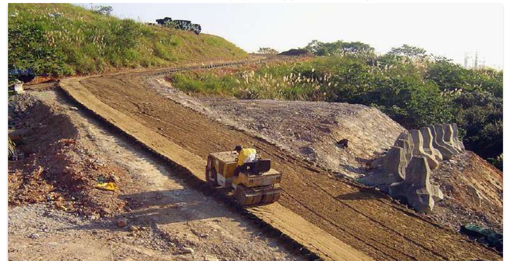
Road reconstruction project using geocell technology
