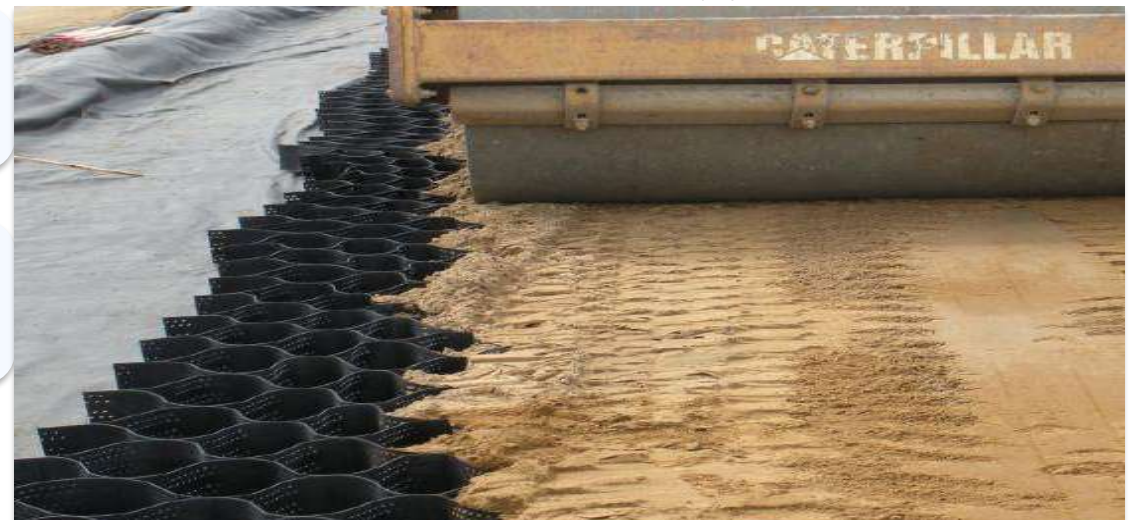
Geocell installation at road construction project site
