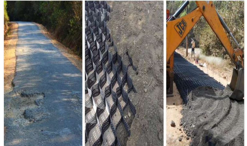
Road reconstruction project using geocell technology
