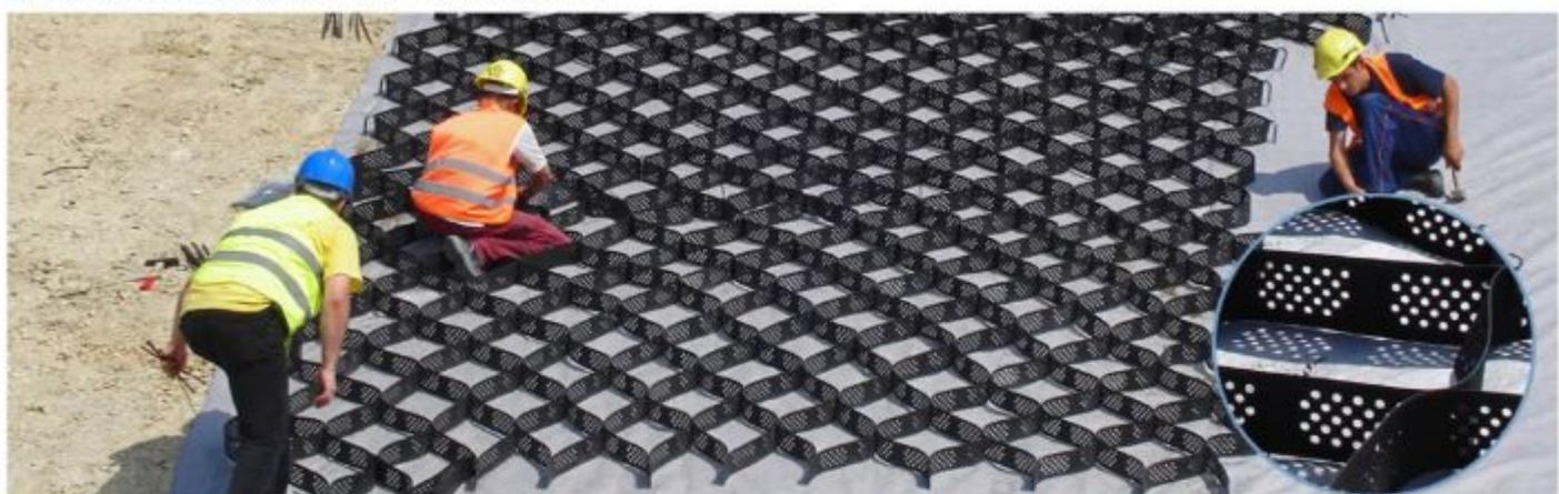
Geocell Is a 3D cellular system. It is expanded on-site to form a honeycomb-like structure which can be filled with sand, soil or other site material. This cost effective solution has multiple applications enabling reduced projects costs and lower environmental impact.
