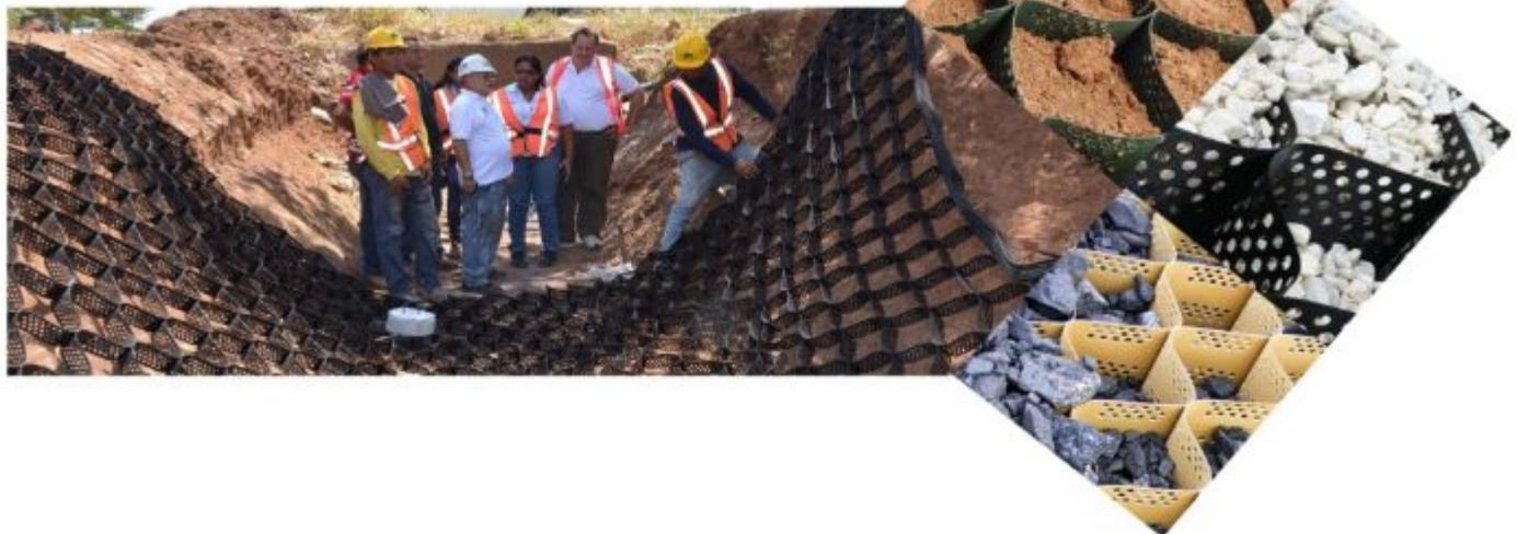
Geocell is usually classified according to the type and structure of the strips (integrated or pierced), their attaching method and the structure of joining points.
